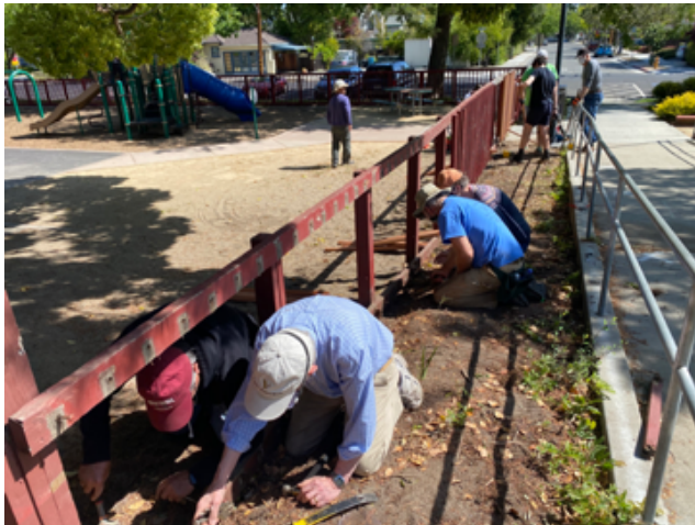
Rebuilding the fence at Bowden Park
