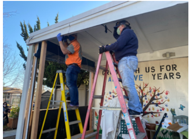
Installing outdoor curtains at Family Connections
