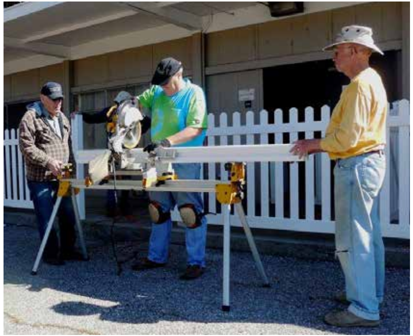
PAKC members went to the East Menlo Park facility of Family Connections to install a new vinyl fence on an outdoor patio. This new fence is next to the vinyl fence we built last Fall, for All Fives Preschool, located in the back of the facility.
