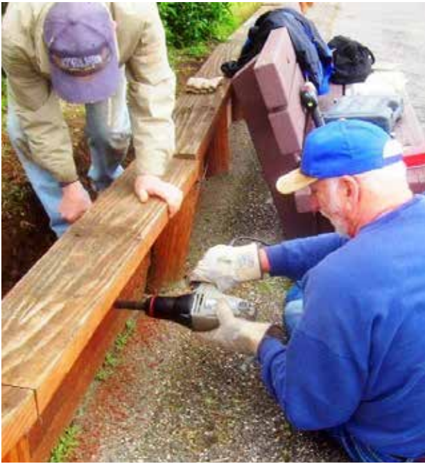
The Club has adopted the Palo Alto Duck Pond as one of our main service projects. Here, a Kiwanian helps to repair a retaining wall.
